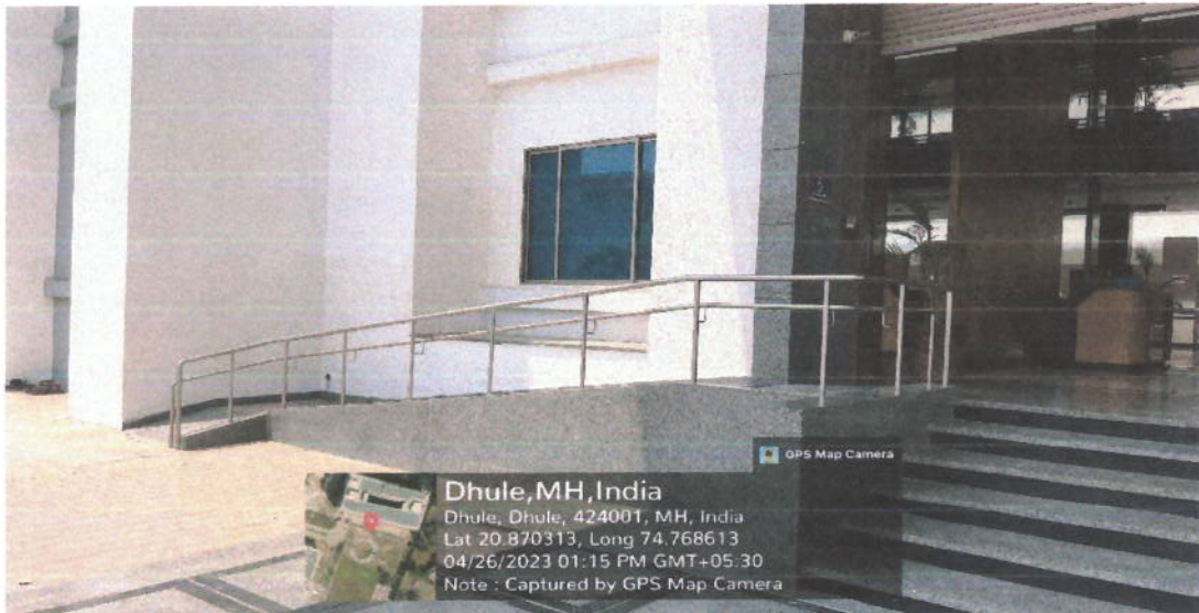
Photo of ramps with railings
